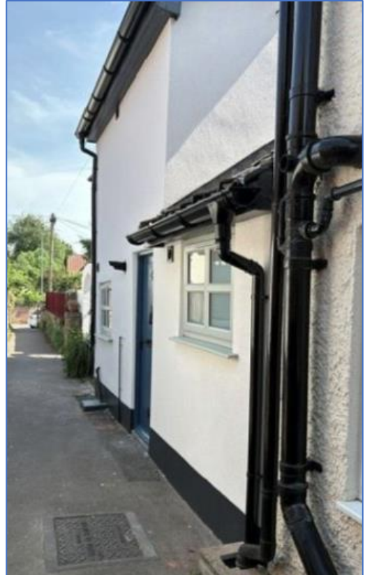
After Photo – Insulation Removed
