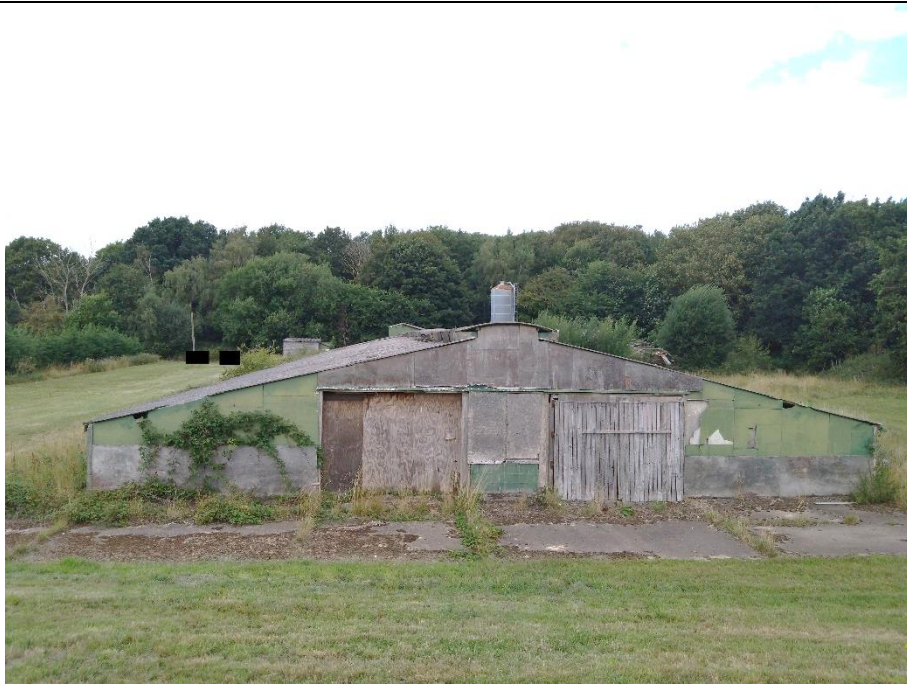
Photo 3 – Southeastern elevation of the longer existing agricultural building
