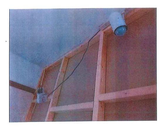
Exposed electrical connections live status not confirmed -Stairwell
