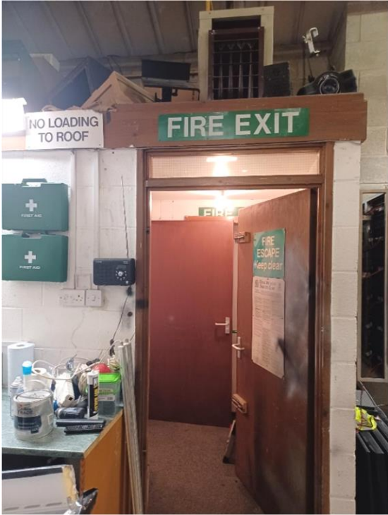
Door to WC
