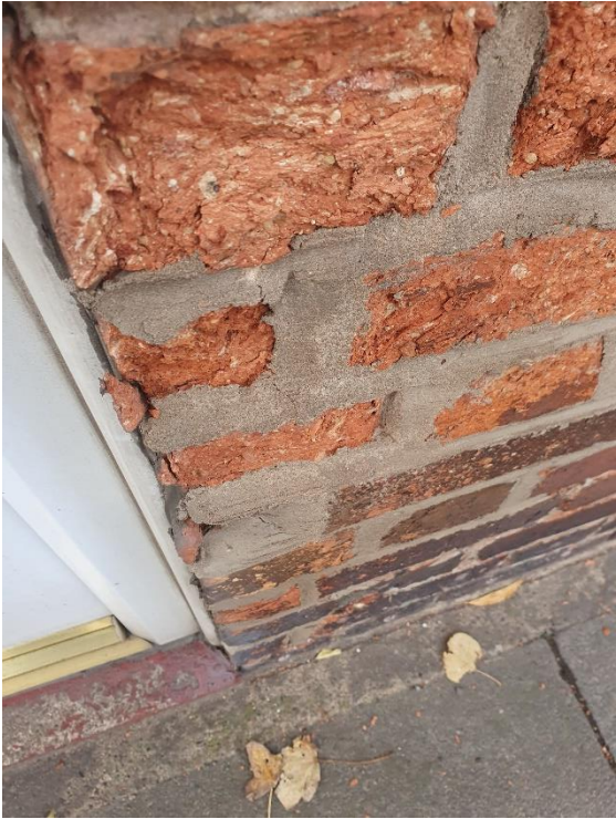
Repairs to front elevation
