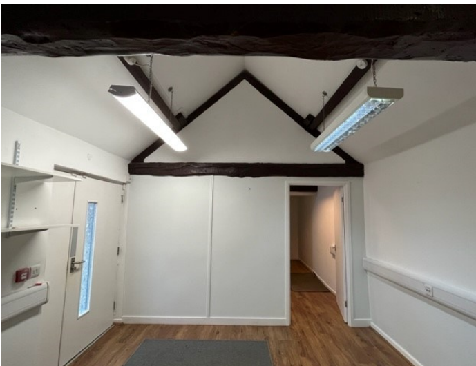
West Wall Internal
