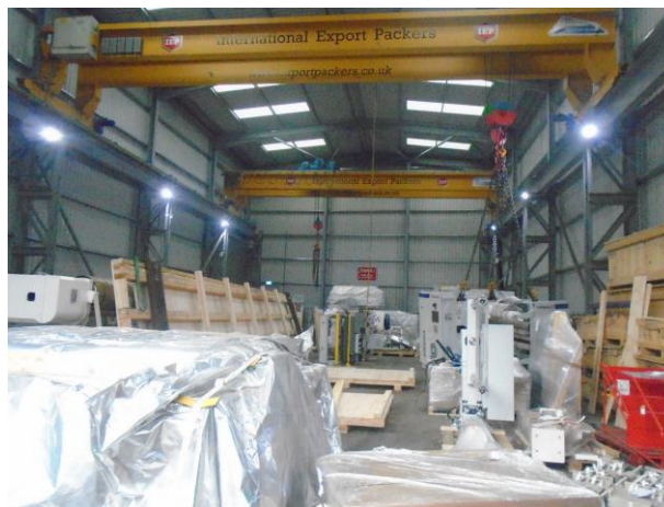
Gantry structure and crane
