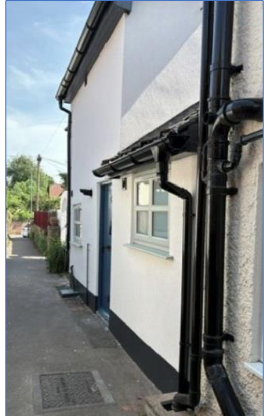
After Photo – Insulation Removed
