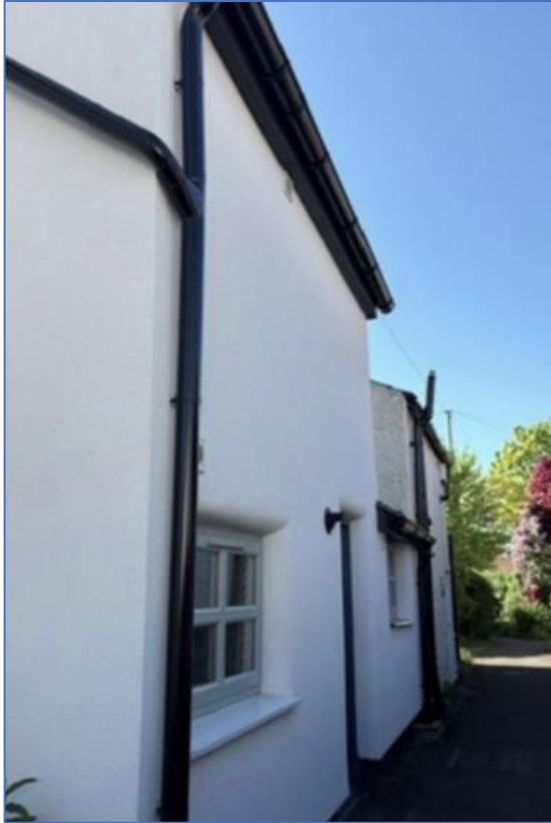
Before Photo – With external Insulation
