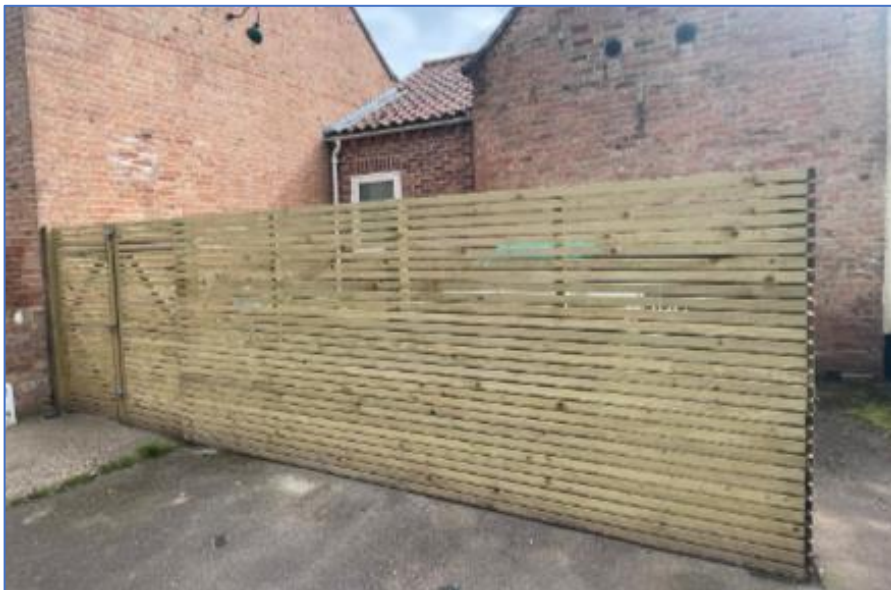
Site Visit Photo – Newly
