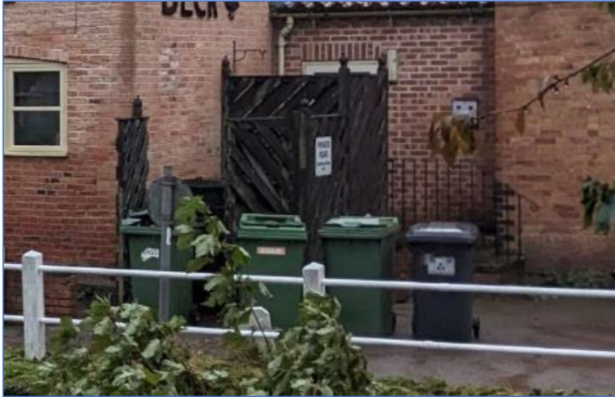
Initial Photo – Taken prior to any recent works
