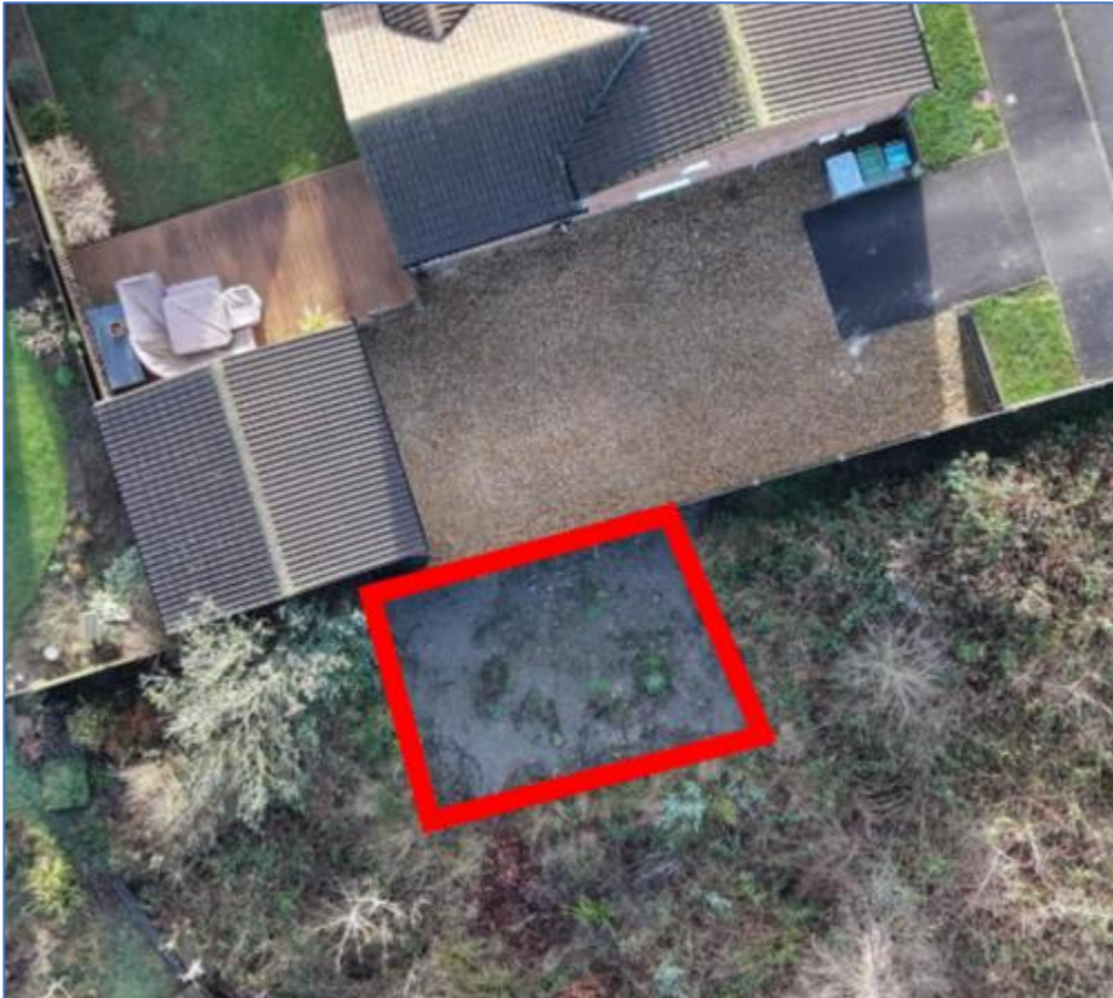
Compliance Drone Photo
