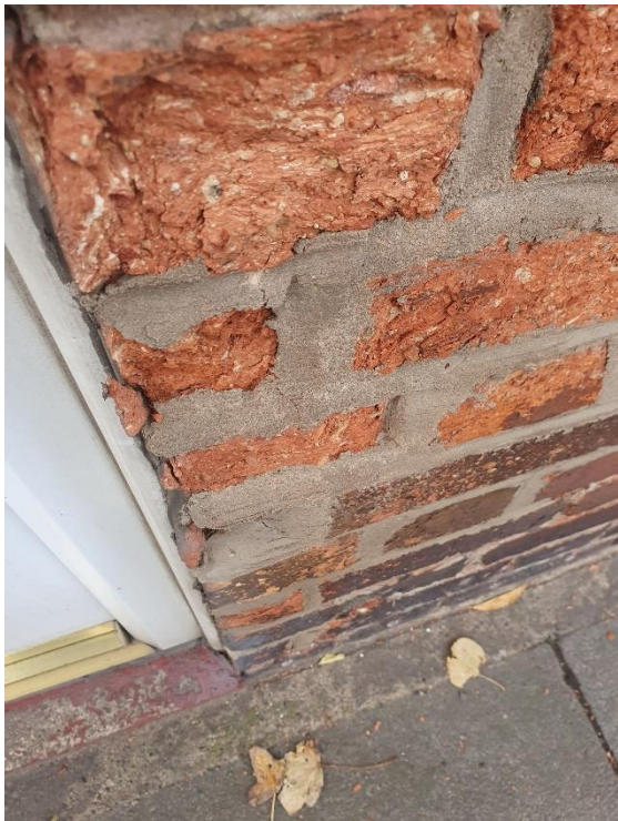
Repairs to front elevation
