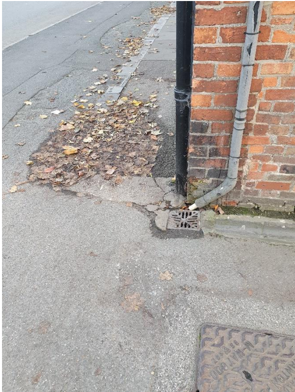
Corner of property where water enters
