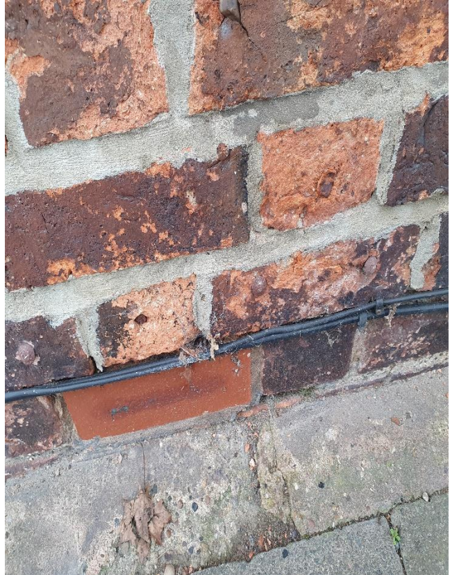
Repairs to front elevation brickwork
